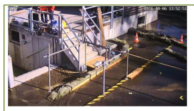
Figure 1: View from camera CAM2 in which channel c3 is visible, as well as the scaffolding holding two radar-based flow measurement systems. The same channel is also visible from camera CAM3.
